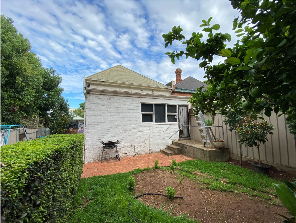
Photo 3.2 – Subject site looking at the rear of the Local heritage place
