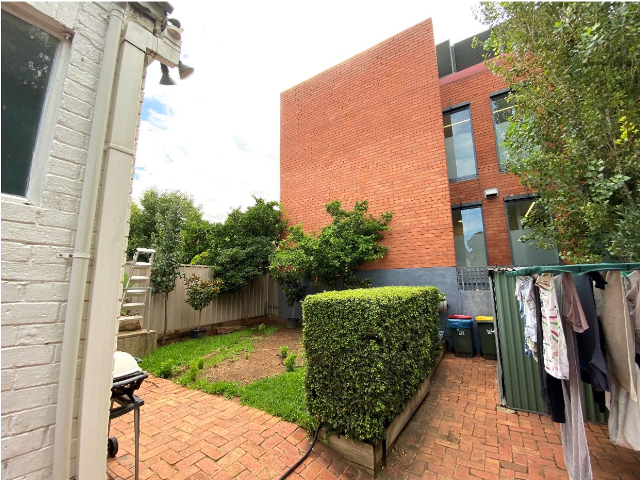
Photo 3.1 – Subject Site with three storey office building at 17-21 Bagot Street
